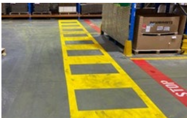
Roadmarking coating applied to concrete warehouse surface. Broadcast aggregate applied to coating for non-skid purpose.
