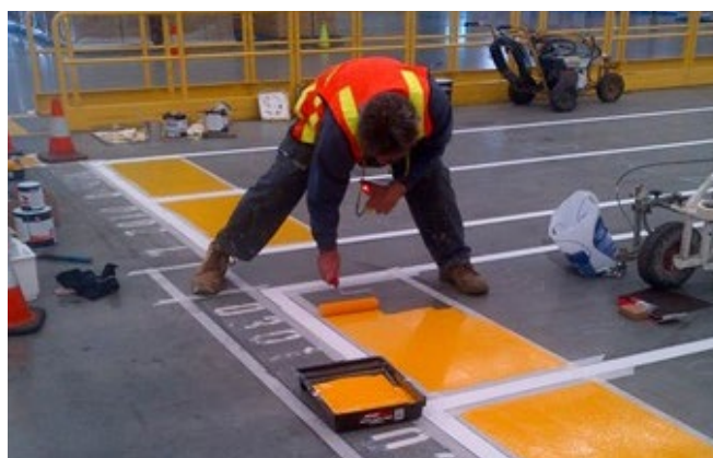
Polyurethane 2-pack coating samples being applied to burnished or polished concrete surfaces to assess adhesion and suitability.
