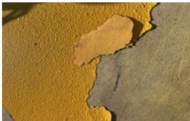
Roadmarking coating applied to external exposed concrete surfaces. Coating applied to wet surfaces resulting in delamination.
