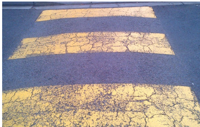
Raised pedestrian crossing coated with Roadmarking coating showing asphalt cracking. Raised surface can increase slip hazard to pedestrians.
