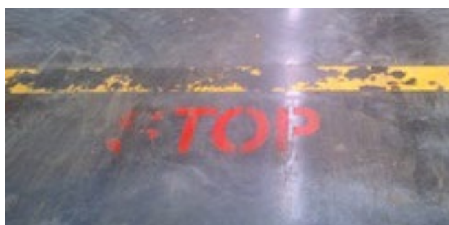
Burnished or polished concrete. Roadmarking coating delamination due to no surface preparation to promote coating adhesion.
