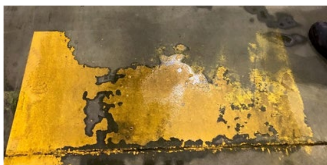
Concrete surface. Roadmarking coating delamination due to poor surface preparation & surface contaminants.
