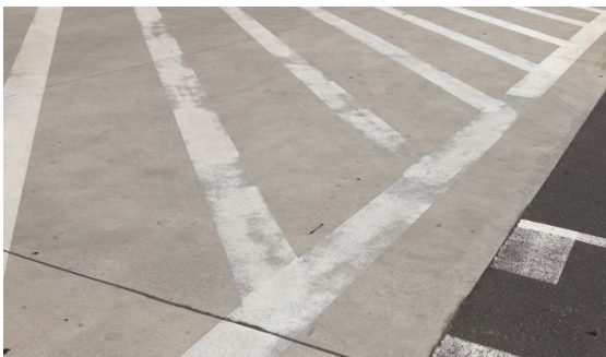
External concrete surfaces. Roadmarking coating wearing away due to no surface preparation prior to application.
