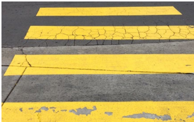
Roadmarking coating applied to both concrete and asphalt surfaces. No surface preparation applied to concrete surface & asphalt cracking highlighted by coating.
