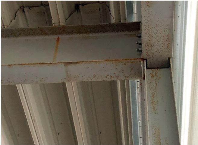
Deteriorated primer surfaces that would require surface preparation prior to applying Dulux FIRETEX® products
