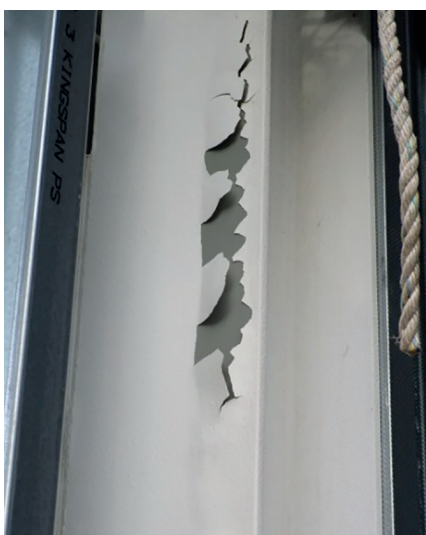
Water damage on external column without topcoat
