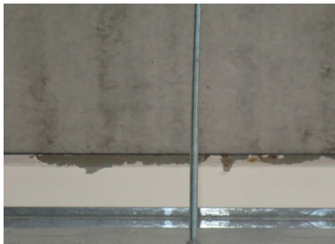
Water damage from concrete slab interface
