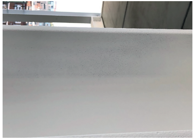
Pin holing and non-closed out coating
