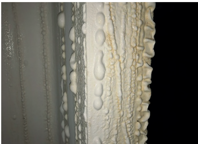
Extreme water damage / absorption
