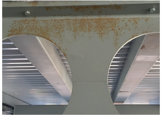
Deteriorated primer surfaces that would require surface preparation prior to applying Dulux FIRETEX® products
