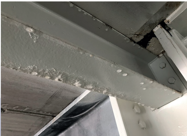
Water damage examples during construction phases
