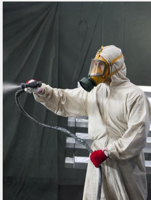
Spraying inorganic zinc silicate primers require a higher level of expertise and experience than zinc-rich epoxies
