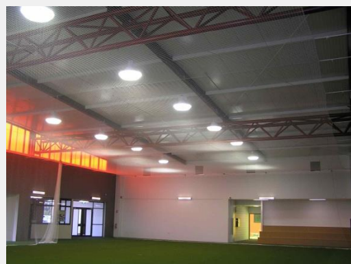
West Tamar Community Centre Training Facility's internal steelwork is primed with Durepon P14
