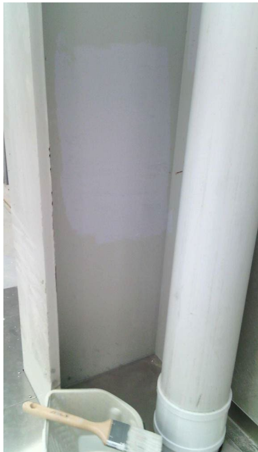
Freshly mixed zinc phosphate epoxy primer was applied over the same product applied only a couple of weeks earlier. Yellowing is clearly visible. As mentioned in the product's data sheet, this yellowing is expected, but will not detract from the protective properties of the product.
