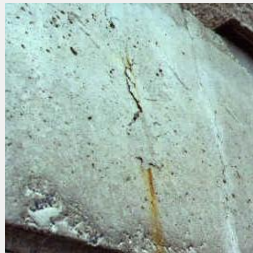
Spots of rust are no reason to panic! They are likely to be due to isolated steel impurities such as chair legs and tie wires, used to space out the steel rebars before the concrete is poured
