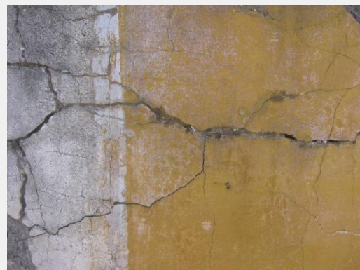
Deep cracks are the first signs of concrete spalling
