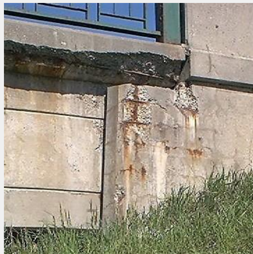
Low concrete cover and no protective coatings gave the rebars no protection from atmospheric acid attack
