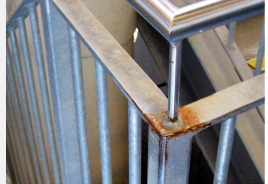
*Etch primers can be used across a range of metals once corrosion and dirt have been removed. Ensure dissimilar metals are isolated from each other to prevent corrosion.*
