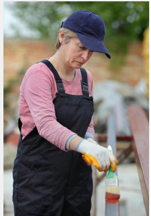
*Whilst the etch primer should be sprayed to ensure a thin, even film, the topcoat can be brushed.*
