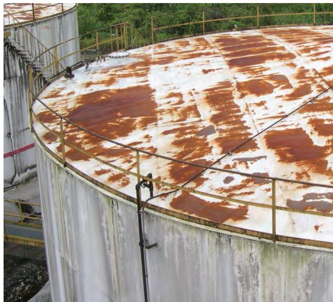
Tanks in PNG. The zinc layer has corroded to white zinc oxide. Red rust shows where the zinc has been completely depleted.
