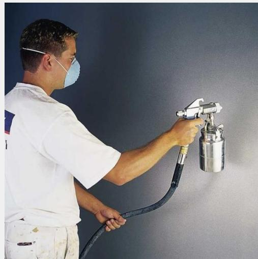
*Applicator is applying a waterborne metallic paint by spray. Polyurethane paint requires far greater PPE, including full positive air-fed head gear.*
