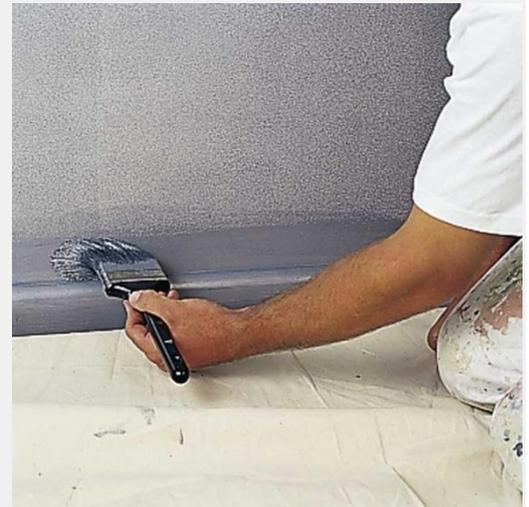
*Cutting in by brush creates a very different appearance compared with surrounding sprayed or rolled areas*
