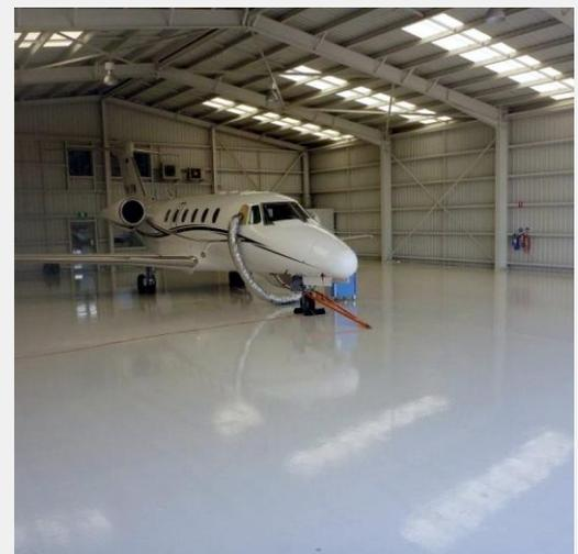
No sign of delamination, grittiness or cracking, so this floor was coated during the specified pot life
