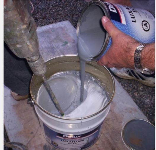
*Some epoxies are very thick and heavy – nothing other than a heavy duty electric mixer can mix these products successfully. Don't try this with a paddle.*
