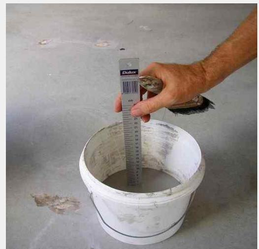
*A measuring stick can be used to measure part kits in the correct proportions –but don't use one as a mixer*
