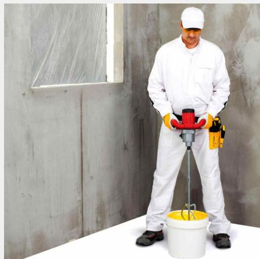
*To mix for a minimum of 3 minutes is made easier with a high speed mixer, a comfortable stance, PPE and a timer –but impossible with a tree branch.*
