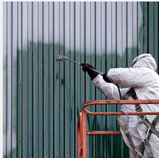
*Acrylic paint is suitable for sheet steel walls*
