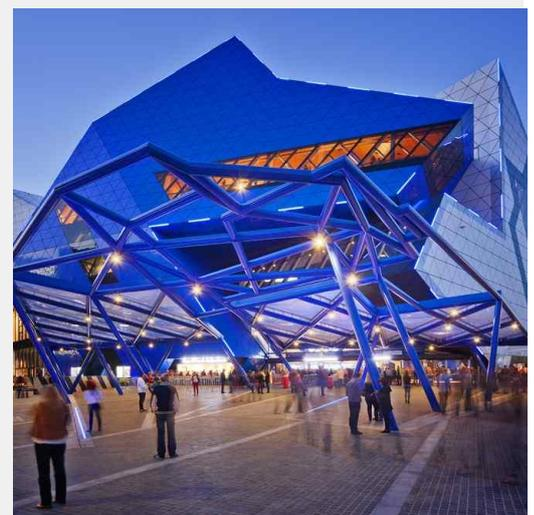
*Perth Arena's perforated aluminium sections are powdercoated in Dulux® Fluorosef®, a very high durability product that is unlikely to need painting for more than 30 years*
