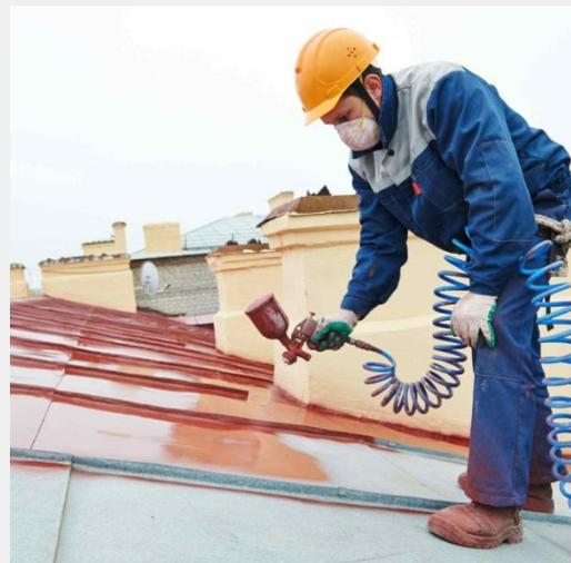
*An acrylic is sprayed directly onto cleaned roofing without primer*
