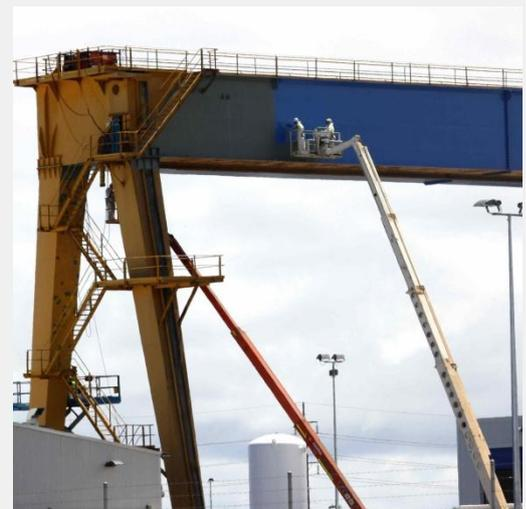
*Goliath mobile crane gets a makeover with **Durebild® STE GF** and **Weathermax® HBR** to extend its service life and minimise future downtime*
