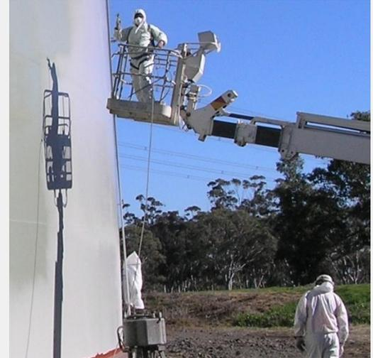
*South Morang Potable Water Tank maintained with **Durebild® STE** and **Weathermax® HBR***
