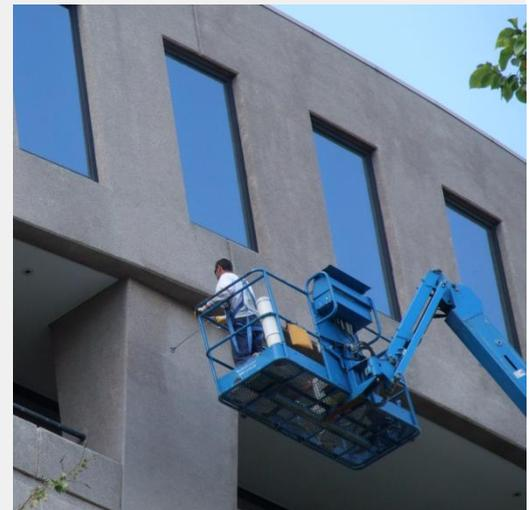
*MLC Melbourne received a thorough water wash before Surfaceshield® HD anti graffiti surface treatment was applied.*
