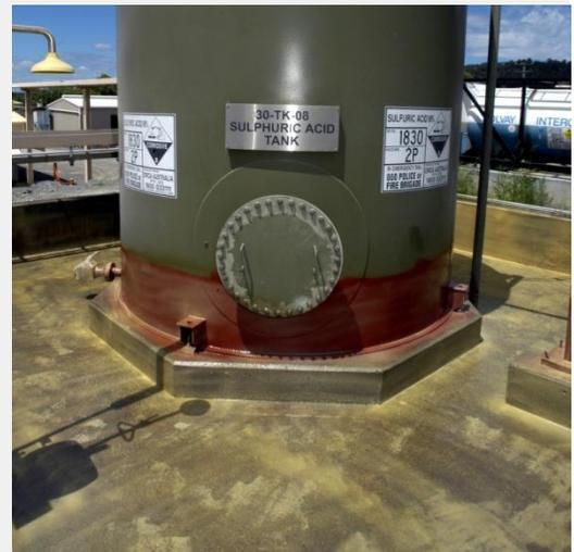
*Highly corrosive sulphuric acid must be kept in bunded areas. Dulux Flexituff<sup>®</sup> Polyurea 's chemical resistance is ideal for lining these bunds*
