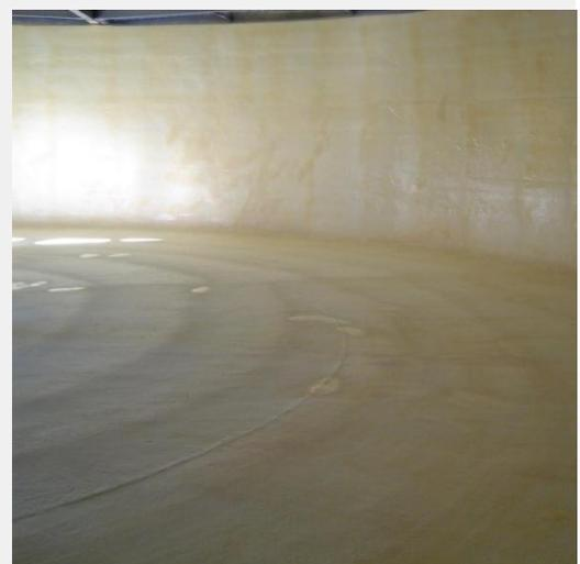
*Dulux Flexituff<sup>®</sup> Polyurea is suitable for potable water*
