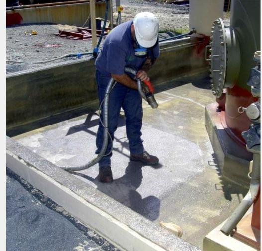
Application OF Dulux Flexituff<sup>®</sup> Polyurea is by plural spray and takes only a few seconds to cure
