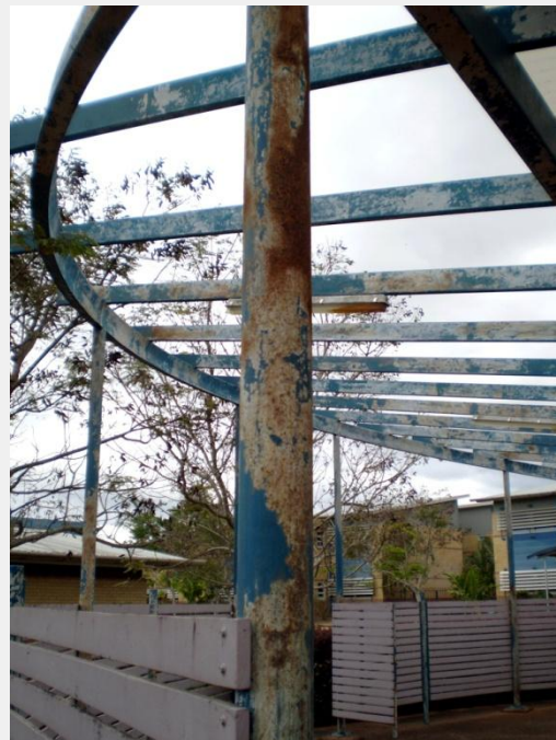
Bentleigh Park Primary School is in a coastal area, and the duplex system failed to stop corrosion of the steelwork
