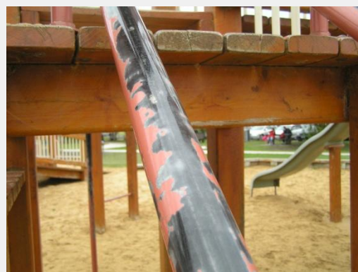
The steelwork of an adventure playground of Lake Pertobe, in Warrnambool, a Victorian coastal town, was coated in a duplex system five years before.
