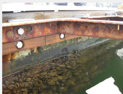
Docklands Landing hot dip galvanised steelwork four years after installation.
