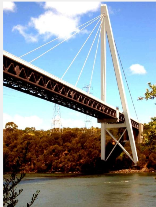
Tasmania's Batman Bridge spans the Tamar River. It won the Engineering Excellence Award in 1968. 75 microns of waterborne inorganic zinc silicate protected the structure without topcoat for 20 years. Only the A frame was top coated and remained maintenance free for 30 years.
