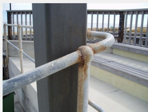
Six year old handrail in a coastal shopping centre
