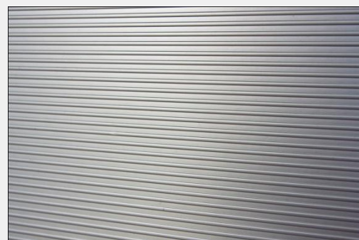
Aluminium and its alloys form a layer of oxide that protects the metal from further corrosion, although in coastal areas aluminium will white rust
