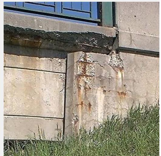
*Low concrete cover and no protective coatings gave the rebars no protection from atmospheric acid attack*
