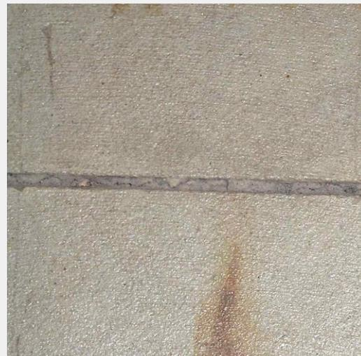
*Well maintained floor joints protect concrete edges and keep the floor level for trolley wheels*
