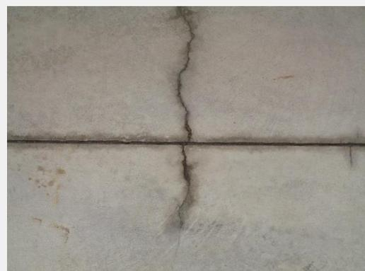
*If the expansion joints don't accommodate sufficient movement, or there are not enough of them, the building will move and create its own joints!*
