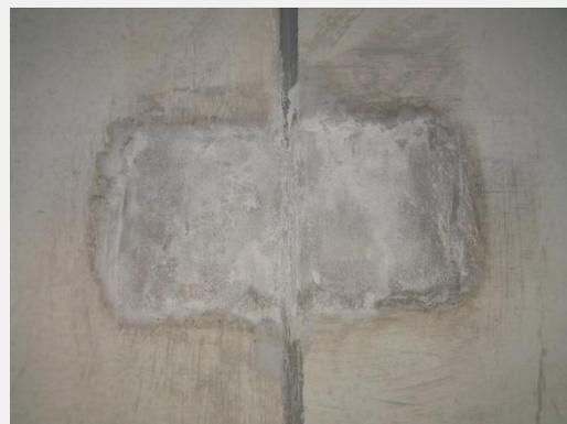
*Repair patch showing laitance*
