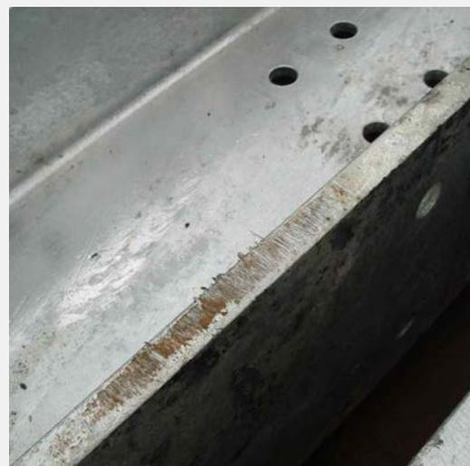
*Excessive abrasion removes the galvanising layer and exposes the steel to corrosion*
