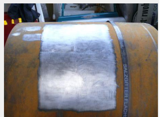
Rust is effectively removed by MBX ® Bristle Blaster ®
