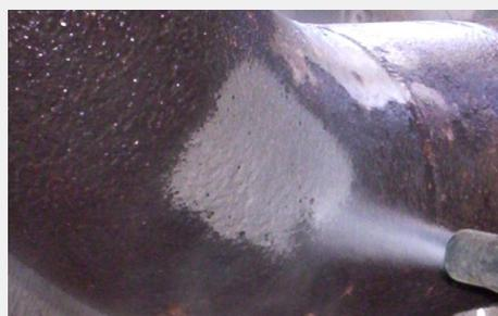
*Wet abrasive blast cleaned steel appears bright and clean, even within the pits*
