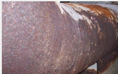
*Widespread rusting and pitting and poorly adhering paint are easily removed by wet abrasive blasting*
