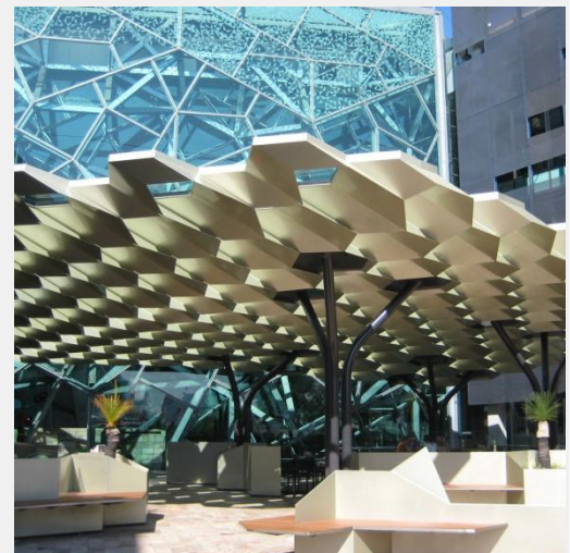
Site welds can be primed and painted on site without loss of aesthetics by skilled applicators
