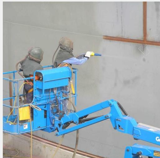
*Spot abrasive blast cleaning is fast and efficient.*
