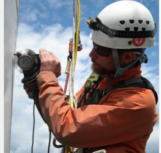
*Bristle blasting is a highly portable and thorough method of removing rust*
