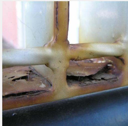
*This photo clearly shows the blue-grey mill scale pushing the coating system off the steel. This catastrophic corrosion began only four years after painting.*
