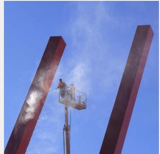
*High pressure water washing was the most practical way of cleaning the CityLink Red Sticks. Abrasive blast cleaning was out of the question!*
