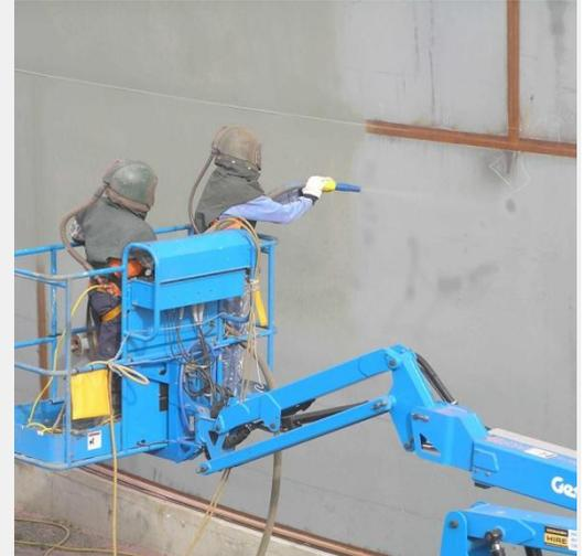
*Spot abrasive blast cleaning is a practical method of removing rust in situ.*
