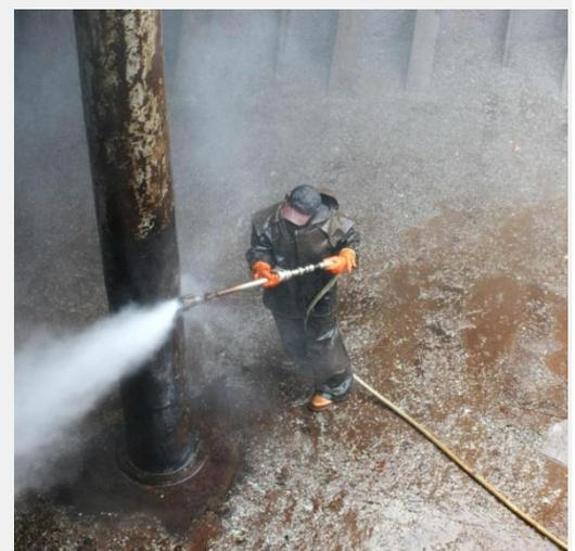
*Ultra high pressure water jet will not create a new profile, but will reveal the original profile of a blast cleaned surface.*
