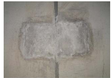
Repair patch showing laitance
